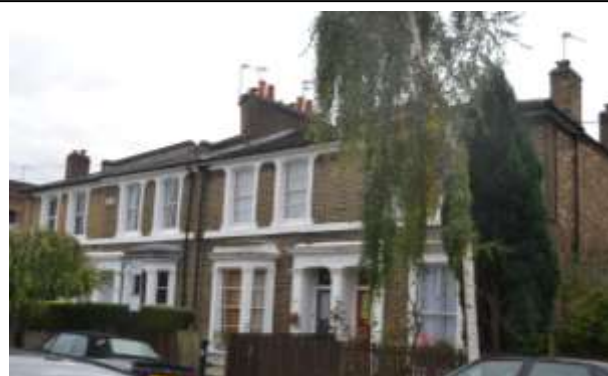
Fig. 5.13 Kent Villas, 1860, Gayhurst Road (formerly Grange Road East)
