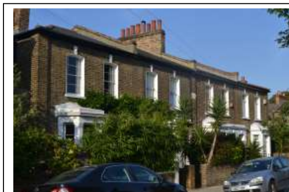
Fig. 5.9 Four-house terrace, Acacia Villas, Gayhurst Road (formerly Grange Road East)
