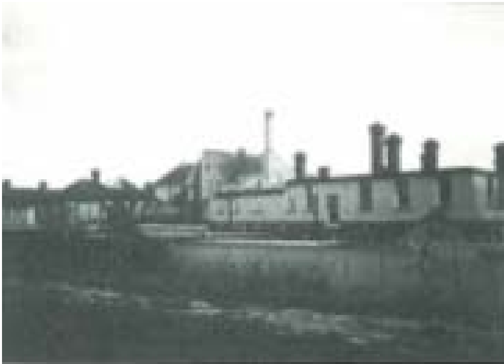
223 and 224. Rooksdown House boarded up. RCM , 1991, p. 9.
