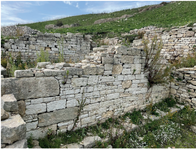
Fig. 6.5: Masonry similar to Soluntum's pseudo-horizontal at Iaitas (photo: Max Peers).
