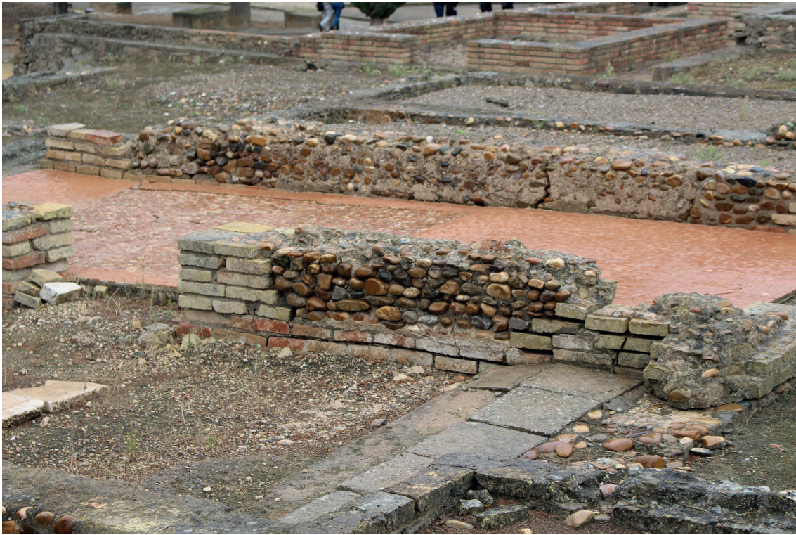
Fig. 5.9: Italica, Casa della Exedra, opus mixtum with pebbles and local bricks (photo: Miko Flohr).
