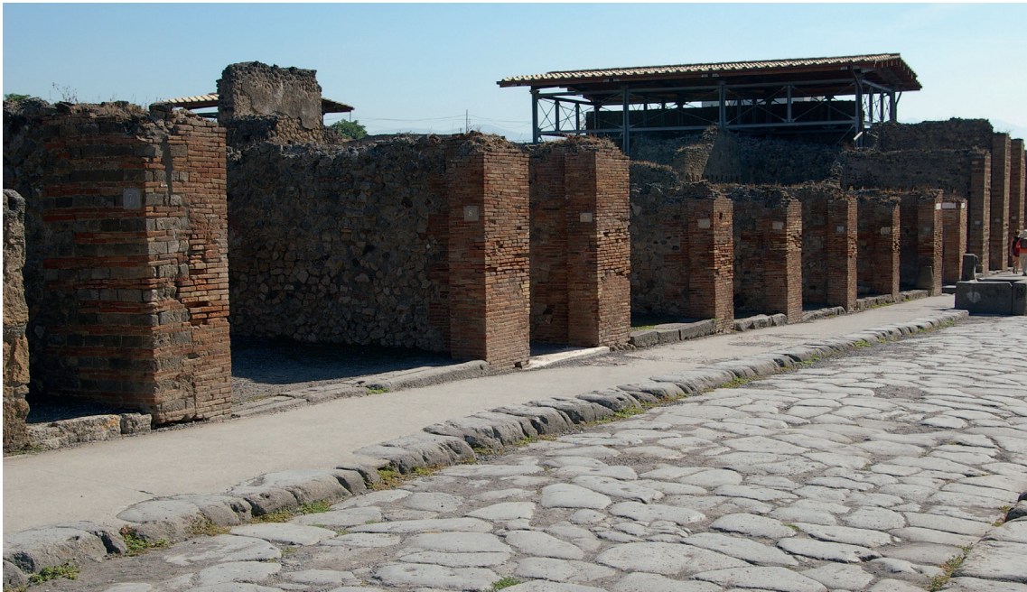
Fig. 5.3: Pompeii, façade along Via dell Abbondanza with mid-1st c. A.D. opus latericium (photo: Miko Flohr).
