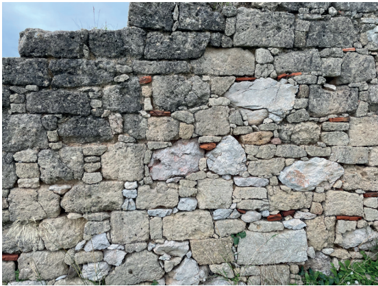
Fig. 6.3: Pseudo-horizontal masonry at Soluntum (photo: Max Peers).
