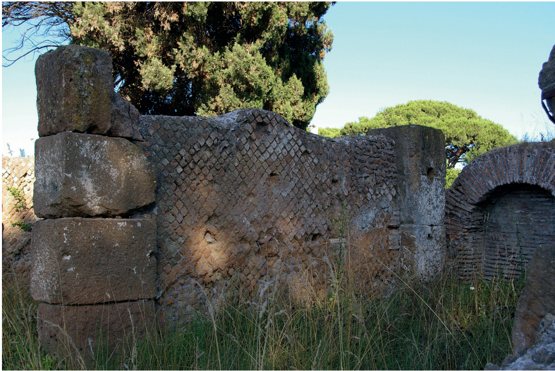
Fig. 5.2: Ostia, so-called Taberne Republicanae (I xi 1), late 1st c. B.C. opus reticulatum in the side-walls (photo: Miko Flohr).
