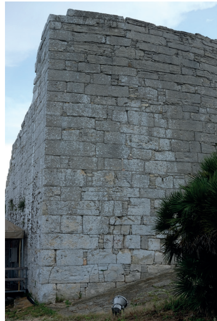
Fig. 6.6: Masonry similar to Soluntum's pseudo-horizontal at Segesta (photo: Max Peers).
