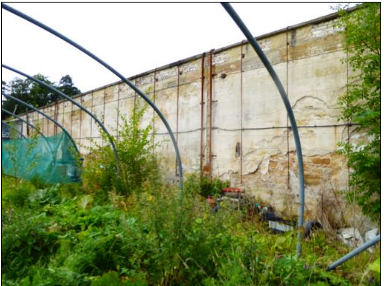
Figure 18. The high south facing wall at Oxenfoord Castle.
