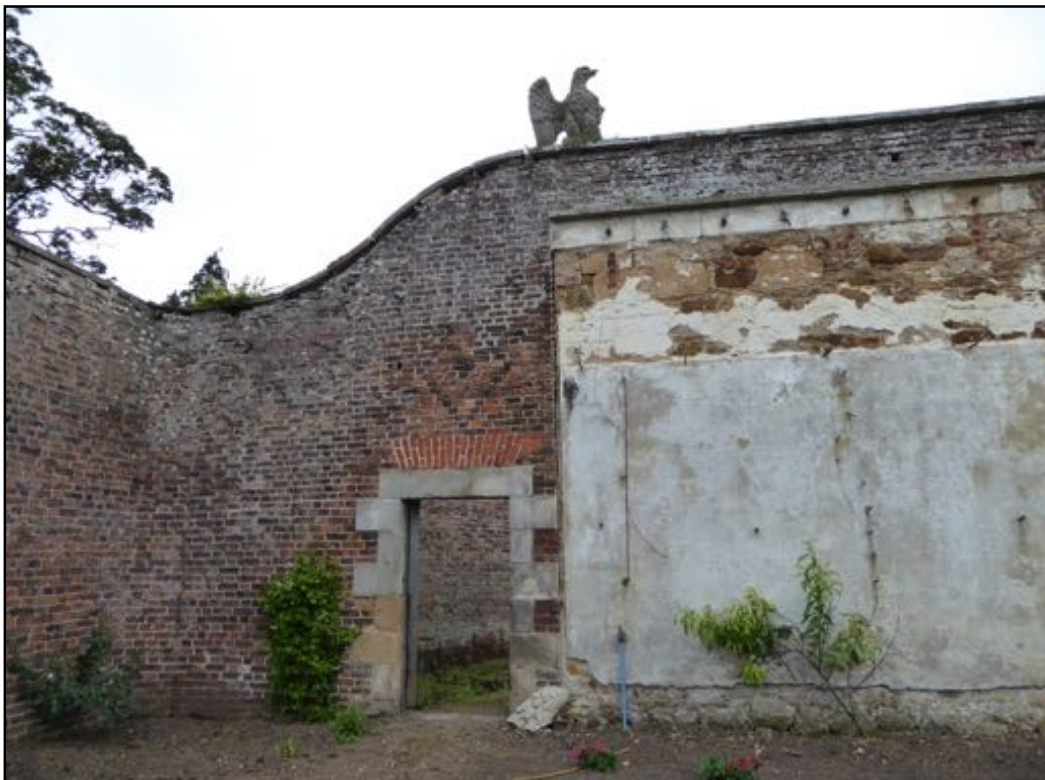
Figure 412. The extant north facing wall indicating where the glasshouses would have been.
