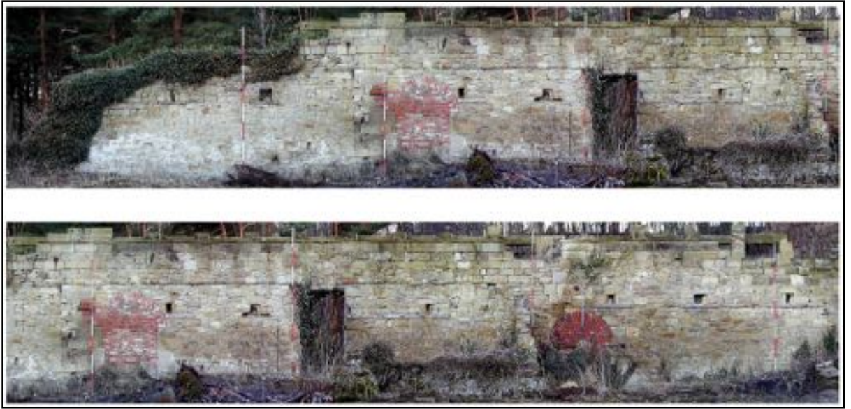
Figure 11. Photographs of the recent excavation of the old walled garden at Alwick, showing the northern hothouse which may have been modified by Hay.
