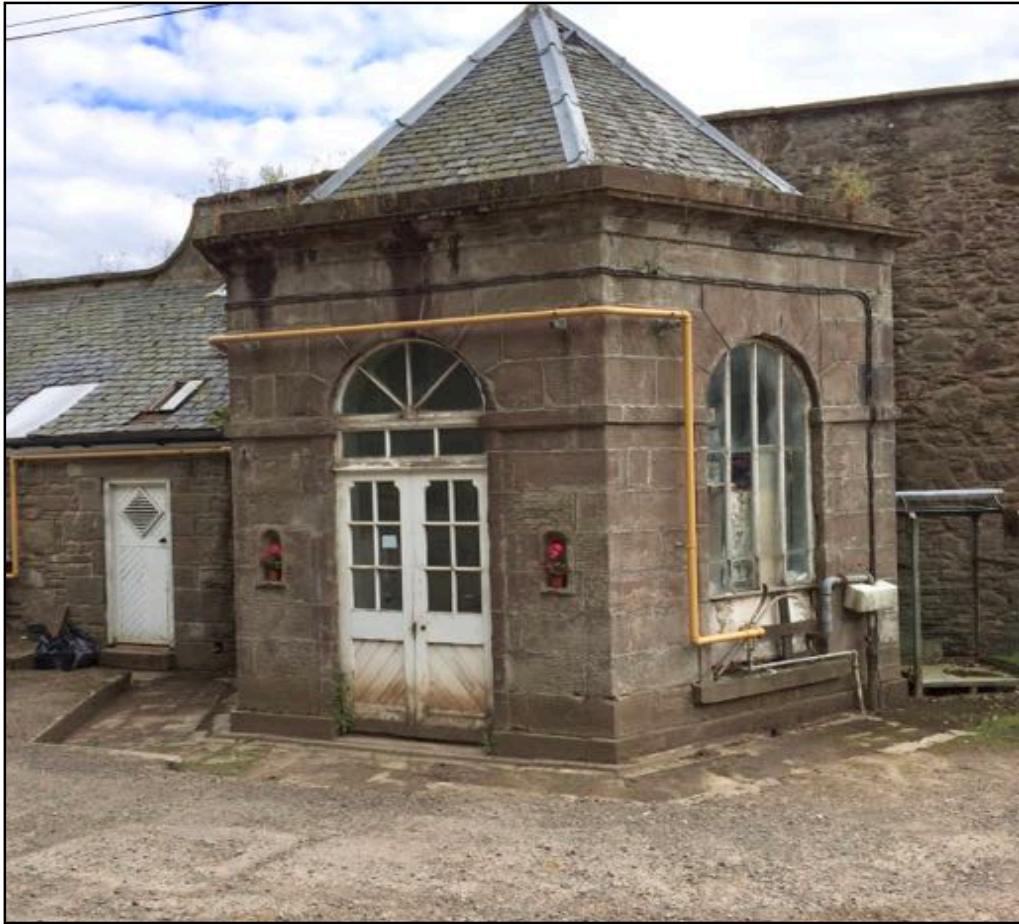
Figure14. Possibly a former orangery. View of one of the back buildings at Camperdown.
