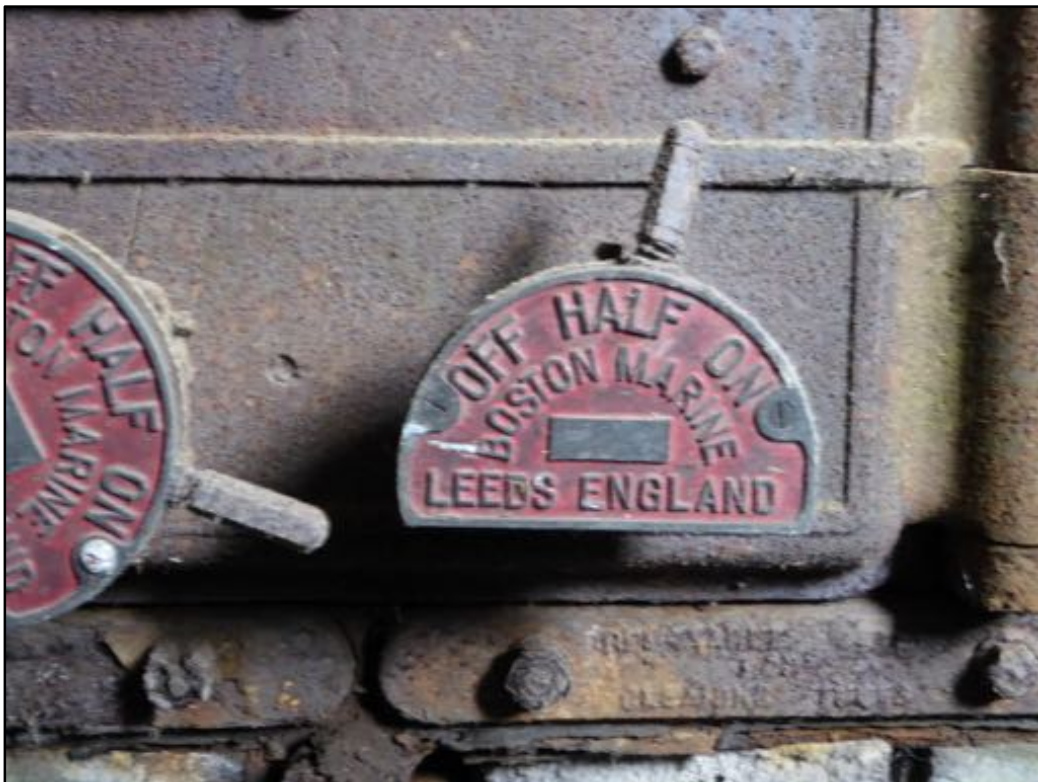
Figure 7. One of the remaining boilers at Prestonhall.
