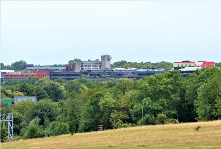
Figure 12: Gateway House seen from Crabtree Plantation (2019).
