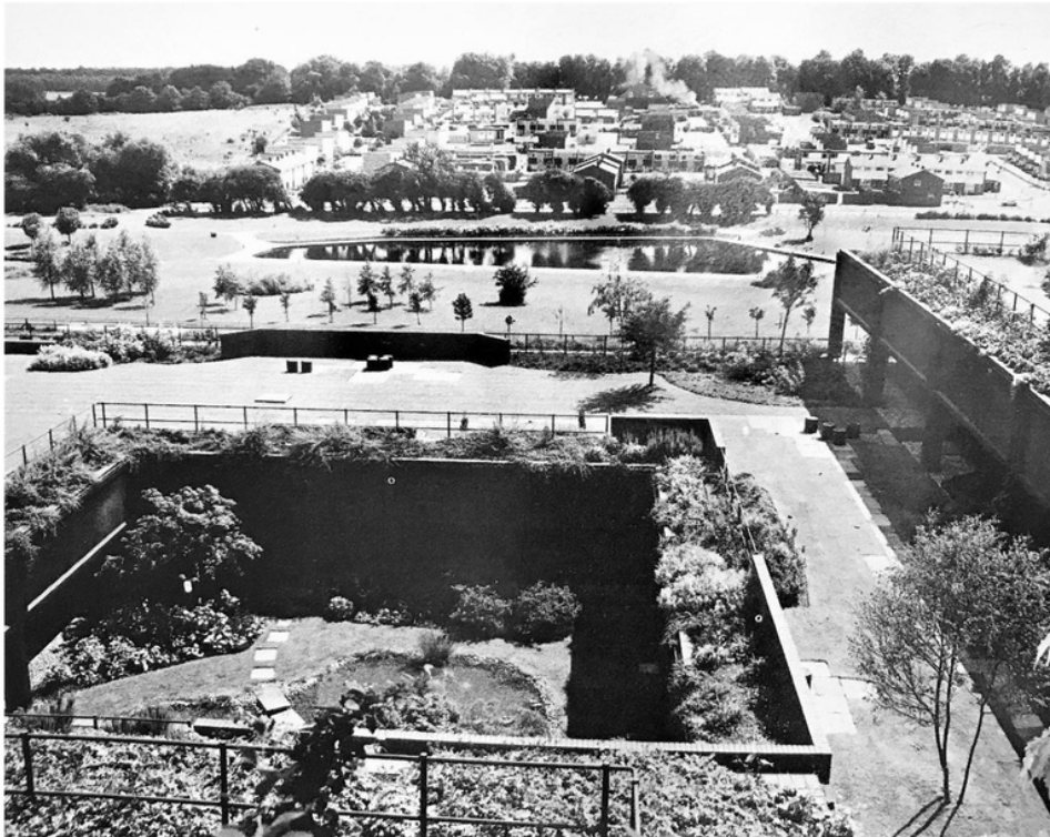
Figure 21: Gateway House, view to the south (c.1977).
