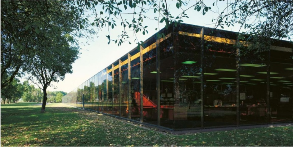
Figure 13: IBM headquarters in Cosham ( undated photograph)
