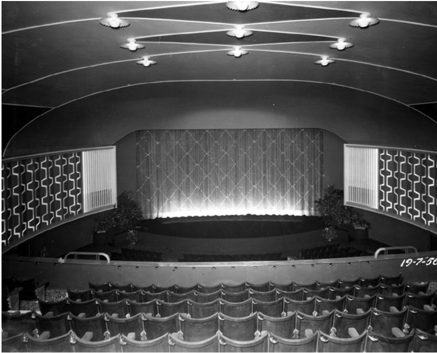
Figure 3.3. Interior of Odeon, Sheffield, July 1956 (Picture Sheffield, Sheffield City Council Archives and Local Studies Service).
