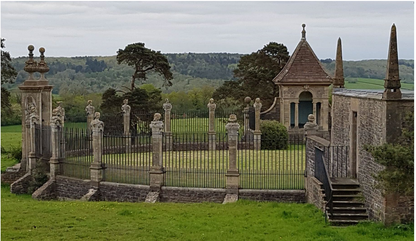
Figure 36. Barrow Court, exedra. Photo: author, 27 April 2022.
