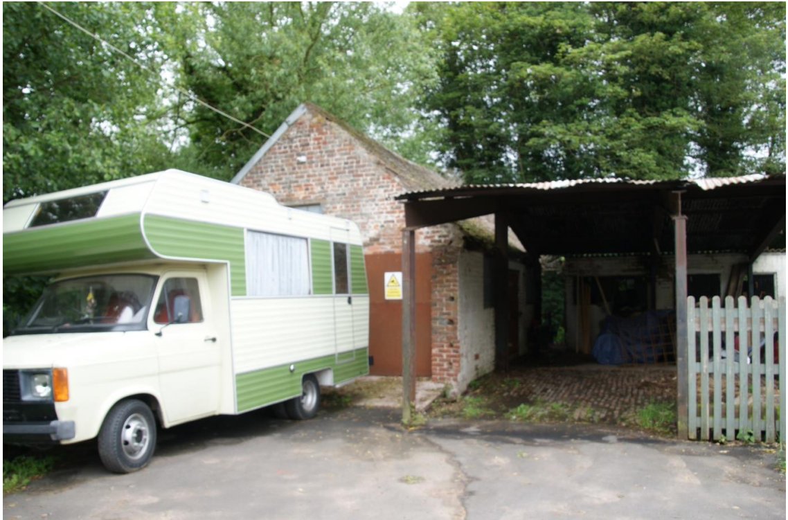
Figure 3.15. The camper van obscures the semi-derelict Hinksford Farm Mill building. The main channel is to the left of the van and runs directly by the side of the building.
