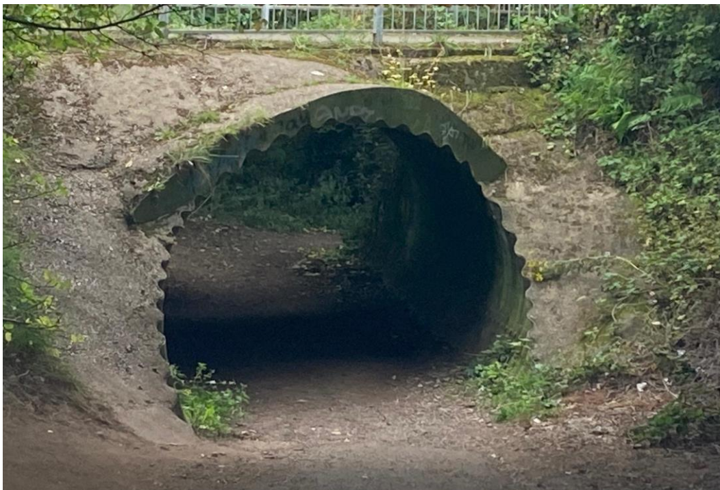
Figure 5.7. The Pensnett Railway was routed through this small bridge near Wombourne.
