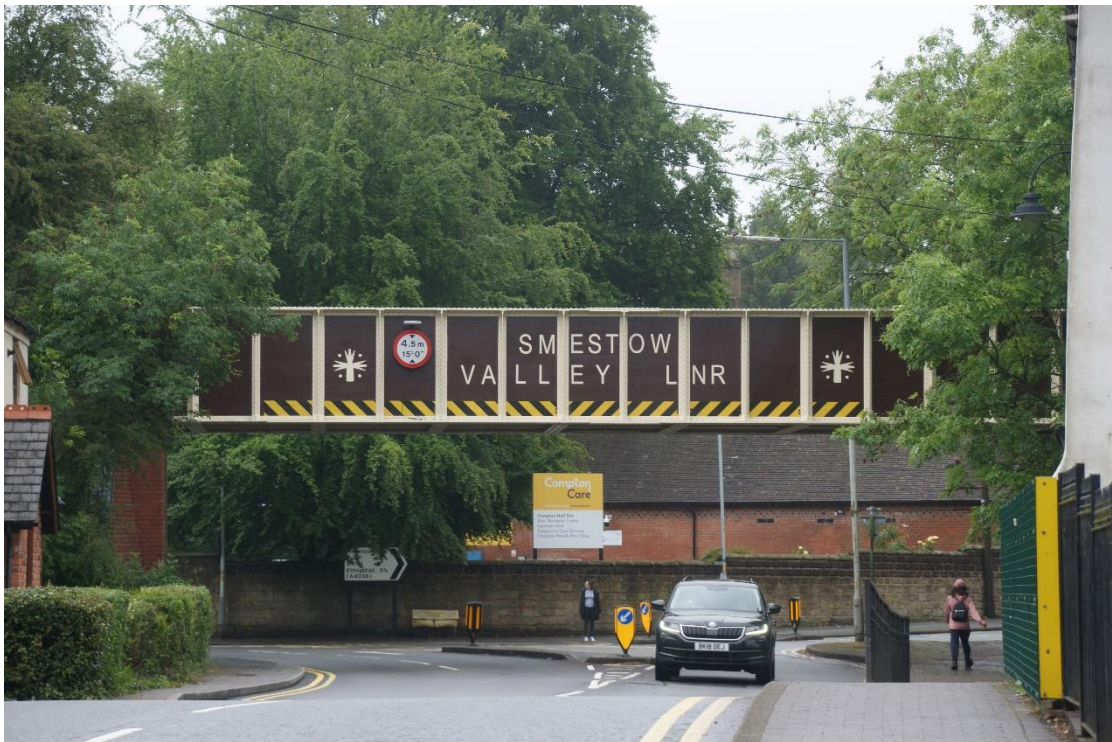
Figure 5.5. The bridge at Compton of the Wombourne railway showing its 1994 conversion to a nature reserve and cycle path.
