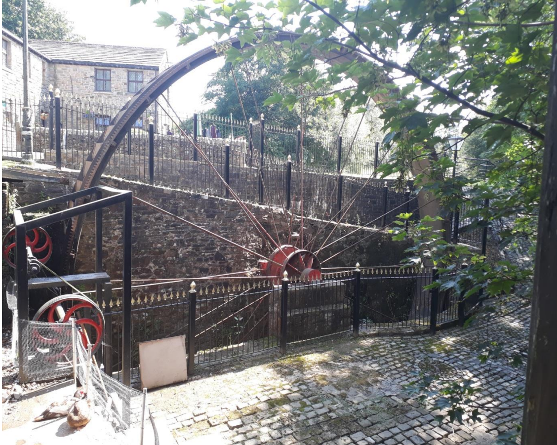
Figure 3.1. Rowarth Little Mill. 9 An example of waterwheel technology from outside the study area demonstrating the peak development of mills. Floods in the 1970s destroyed the mill but left the 24' diameter wheel intact, in its original location. The wheel is mid-shot, fed by a trough. The mill building was where the photographer is standing.
