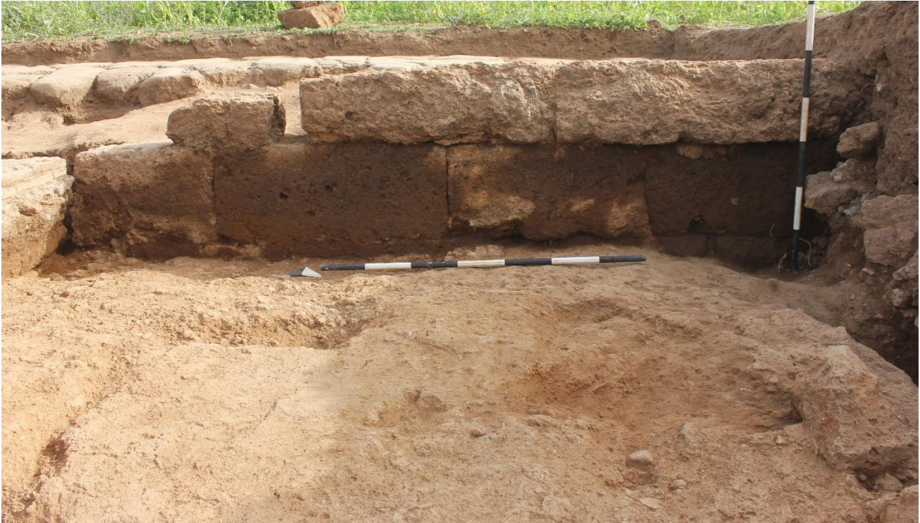
Fig. 23. Rear wall of tabernae in Room V.3 showing tuff ashlar construction, viewed from south.
