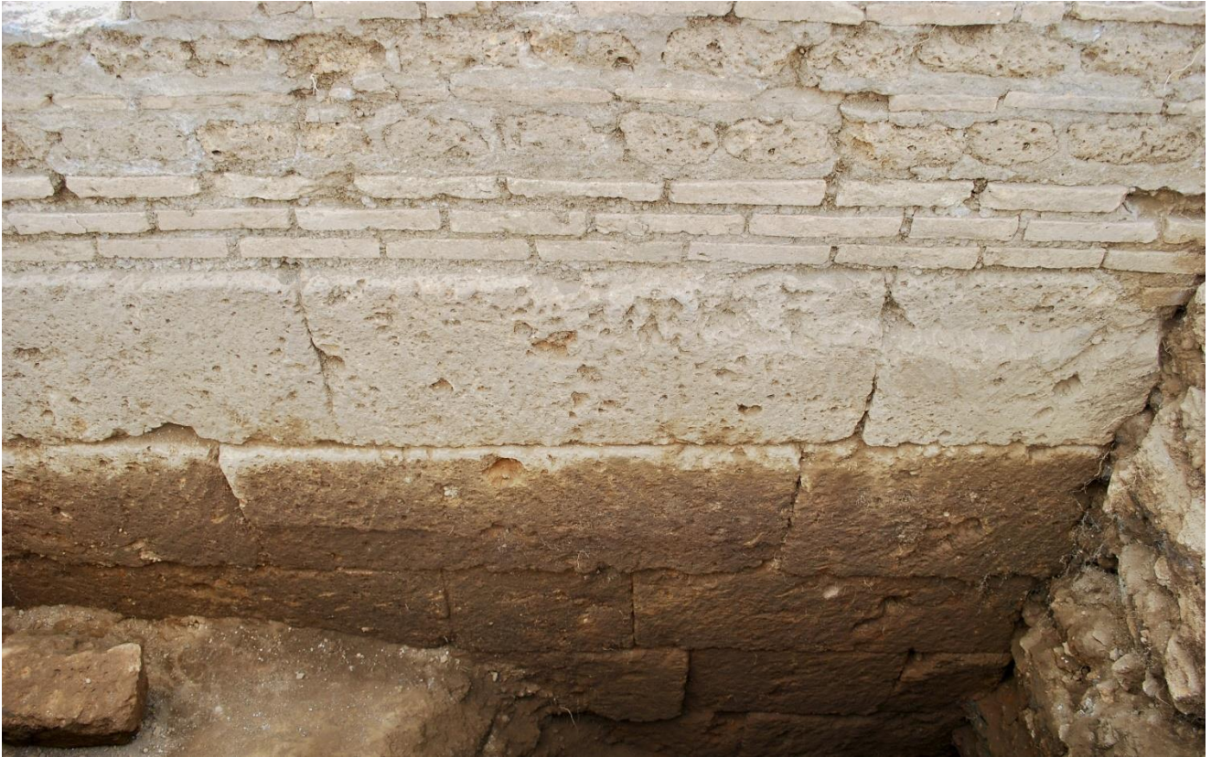
Fig. 4. Wall of central corridor of macellum's northern entrance showing deep foundations of ashlar superimposed by opus vittatum.
